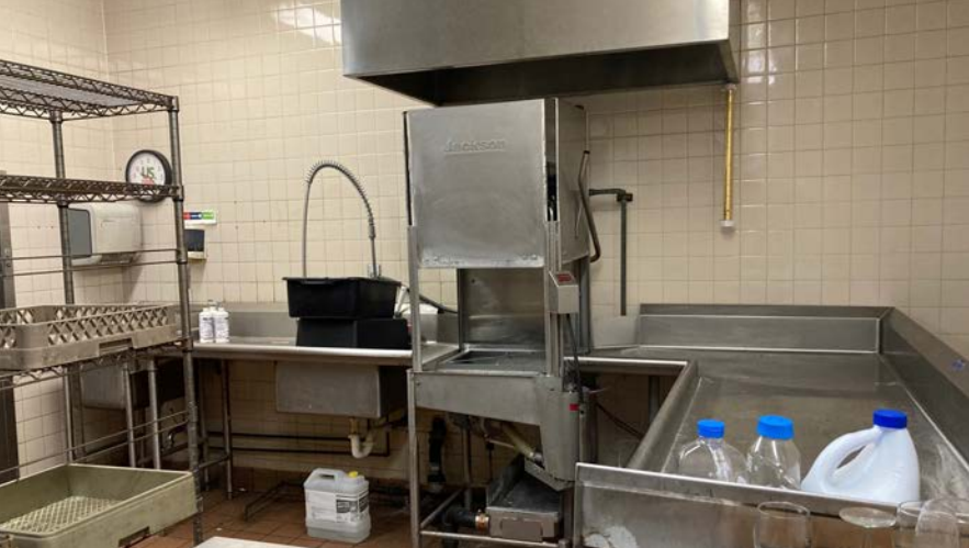
Hood Already Installed
