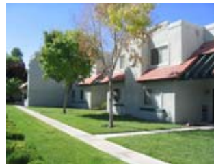
CharterMac has provided an $11.2 million loan for the 168-unit Heritage Pointe Apartments in Henderson, Nev.
